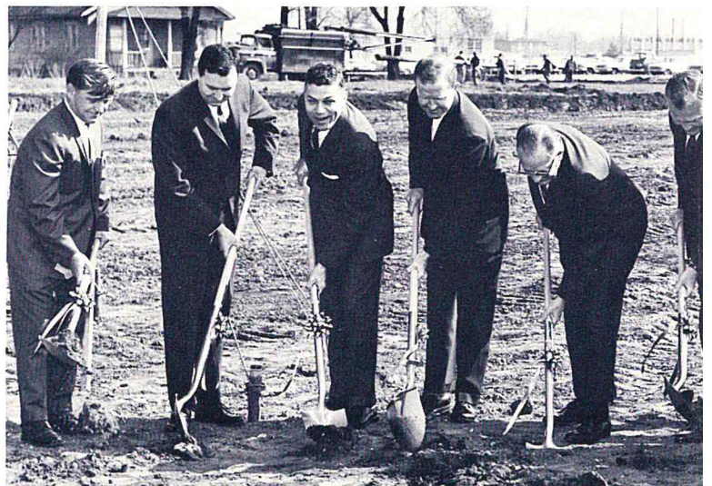
Other officials join President Connaughton and Dr. Carmichael in groundbreak
